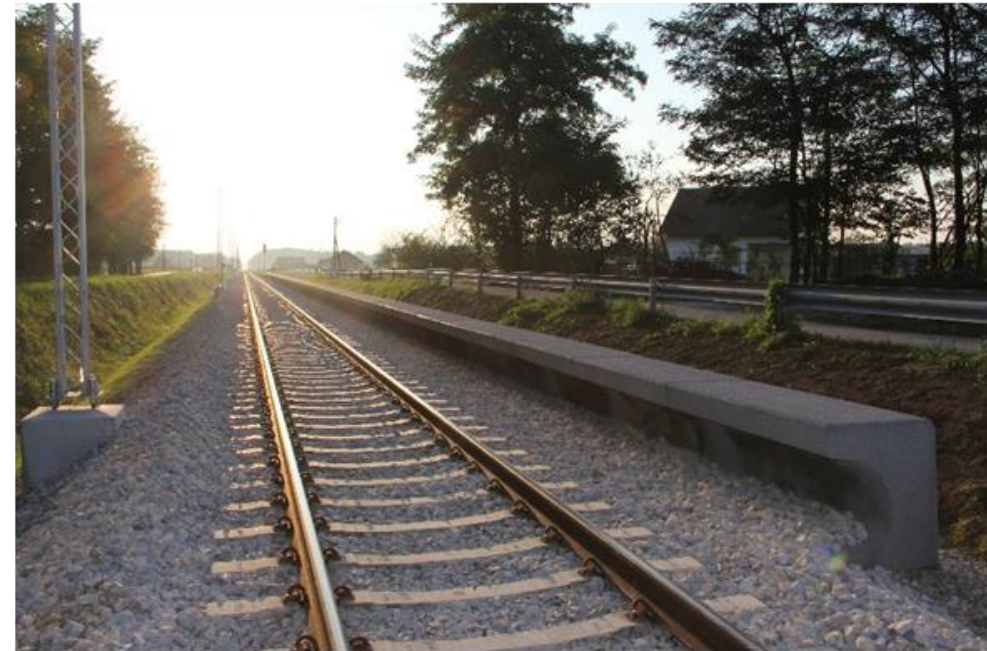
Absorbing surface (single-grain concrete)
