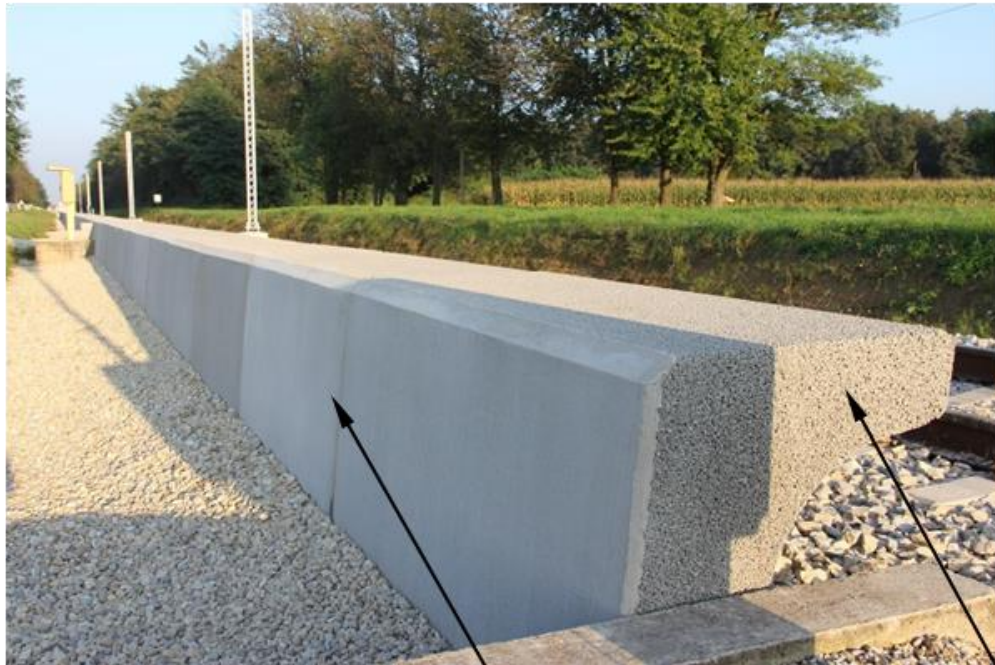
Insulation surface (closed standard concrete with brush-stroke structure)
